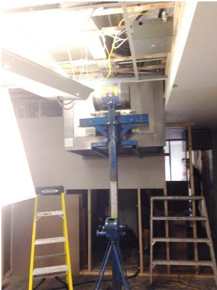
This past week, Quest Metalwork has delivered and installed the ductwork for the venting. The large (500 lb.) range hood that we have been waiting on for over a month was delivered and installed Friday October 28. Hallelujah!
